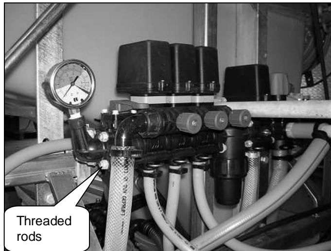
Electric Control Unit
